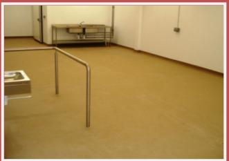
NIFL Resin Flooring successfully installed 1,500m<sup>2</sup> of Altropol Polymer Modified Granolithic Screed and Altrocrete PU HF Heavy Duty Polyurethane Screed to the Leeming Bar Food Enterprise Centre.
